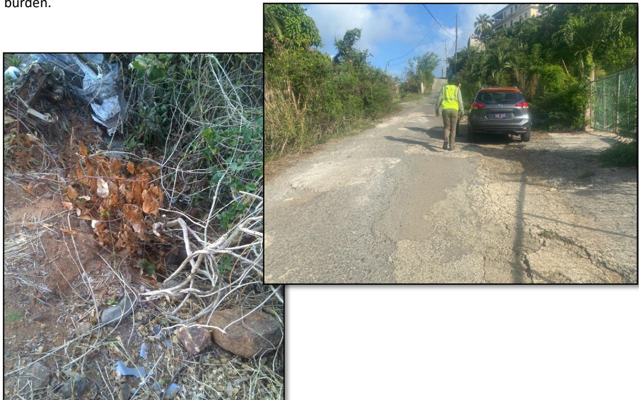
Figure 36. Culvert inlet plugged by sediment (left) and roadway erosion (right).
